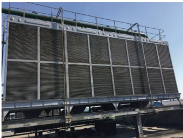
Tongxiang site Variable Speed Driver on big motors to save energy
