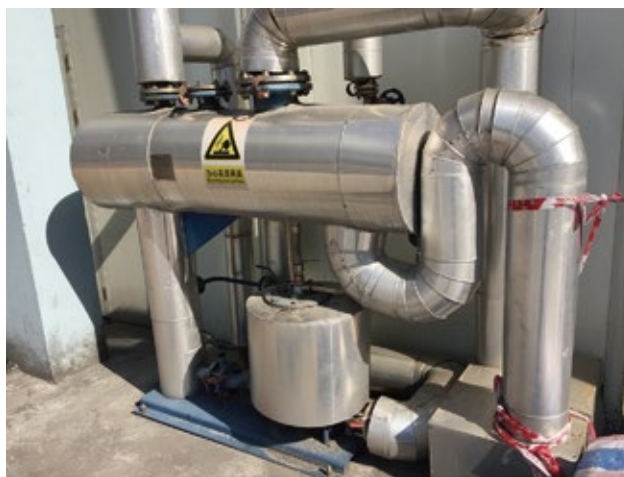
Tongxiang site waste heat recovery
