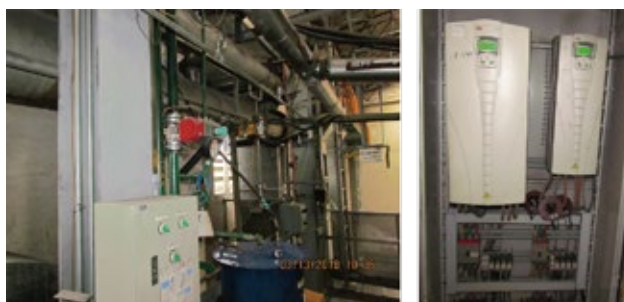
Shunde Variable Speed Driver on pumps to save energy
